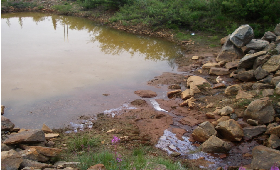
Photo D Seepage from toe of dam into seepage pond
