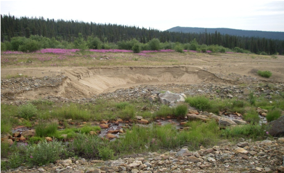
Photo L Slope Failure on Combined Spillway
