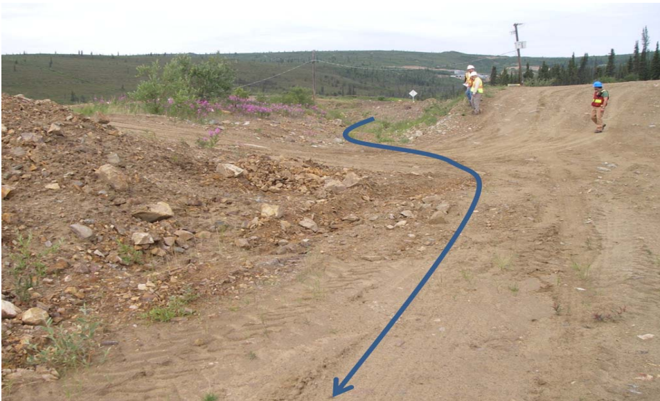
Photo K Emergency Spillway Channel at Access Road Crossing
